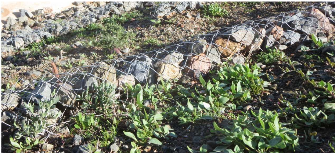
Figure 29. Seedlings germinating on a slope stabilized with stone-filled wire mesh “Potch sausages”
