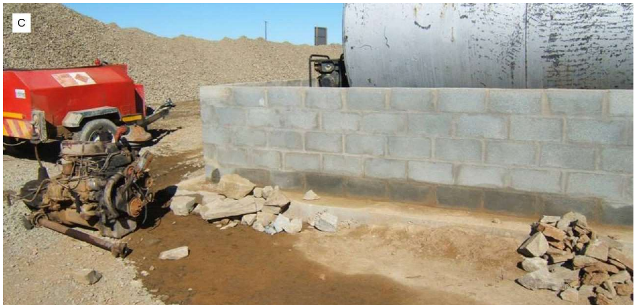
Figure 23. Pollution caused by a diesel spill from a bunker.
