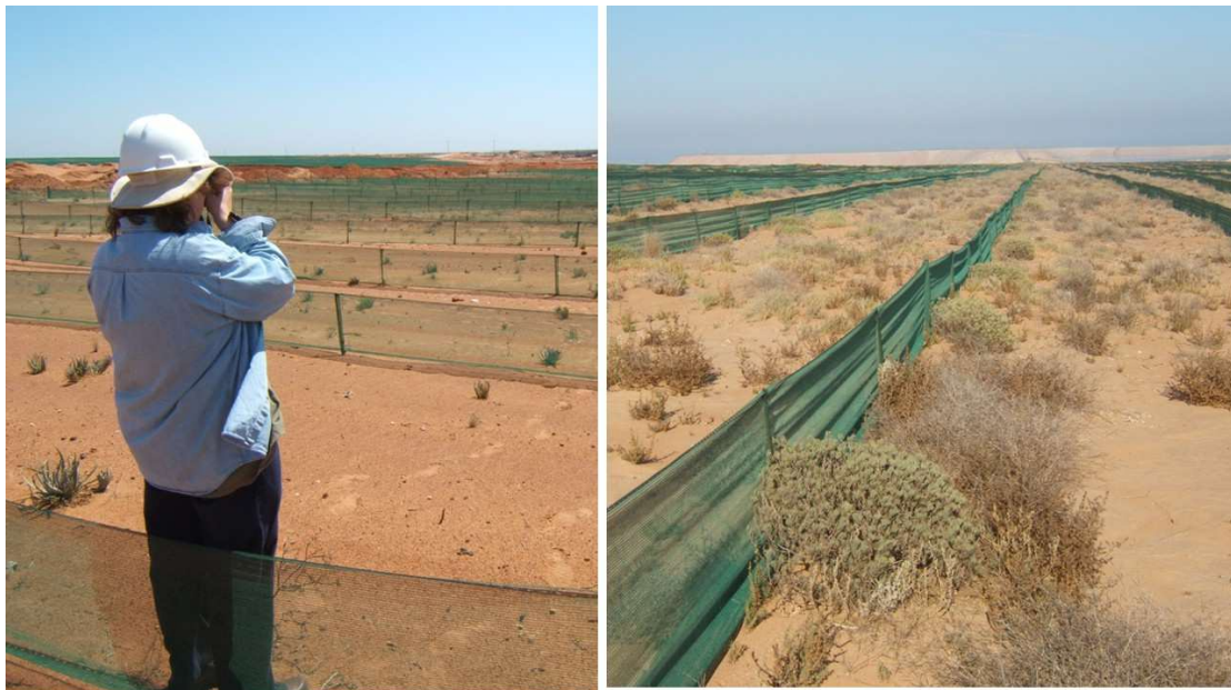
Figure 25. Wind netting at Namaqua Sands mineral sands mine on the coast of Namaqualand in Succulent Karoo
