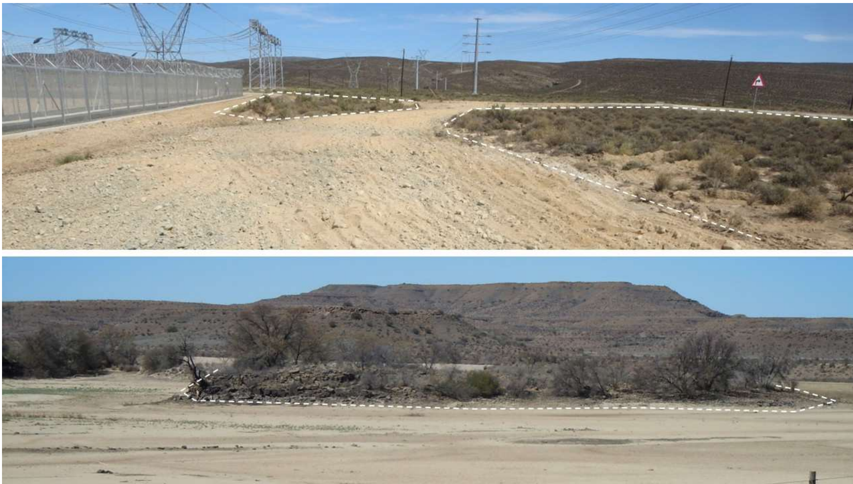
Figure 20. Islands of natural vegetation retained on a construction site and in a borrow pit
